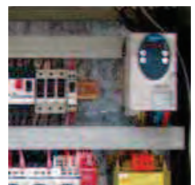
Speed regulation through inverter with digital display.
